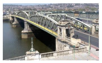
NEC4 Engineering and Construction Contracts were used to refurbish an iconic set of three bridges over the River Medway estuary in Rochester, southeast England. The £12 million project included strengthening, repairing, painting, waterproofing and resurfacing the 140 m long steel bridge decks as well as replacing parapets and expansion joints and repairing the cast-iron, masonry and concrete piers.
