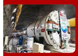
Assembly of TBM inside the Tunnel
