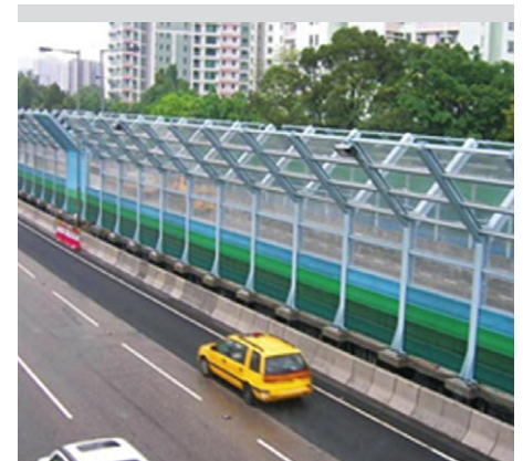
Noise barriers on Fanling Highway, using NEC3 ECC Option C
