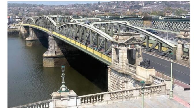
NEC4 Engineering and Construction Contracts were used to refurbish an iconic set of three bridges over the River Medway estuary in Rochester, south-east England. The £12 million project included strengthening, repairing, painting, waterproofing and resurfacing the 140 m long steel bridge decks as well as replacing parapets and expansion joints and repairing the cast-iron, masonry and concrete piers.
