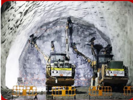
Drilling blast holes on blasting face
