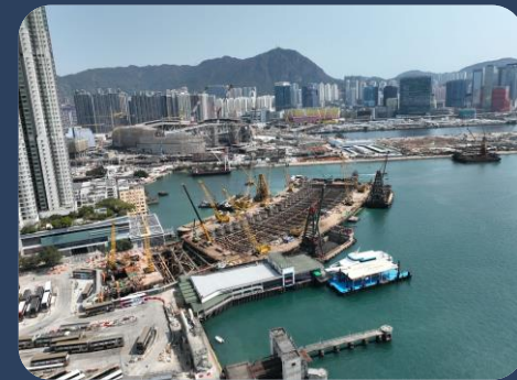
Construction of temporary marine platform and cofferdam for underwater tunnel
