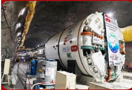
Assembly of TBM inside the Tunnel
