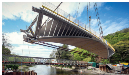
The 40 m long, 300 t stainless-steel and concrete composite structure was installed in a single lift
